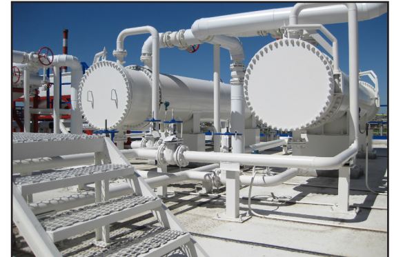
All nut bolts coated with Chesterton 785 Parting Lubricant.
