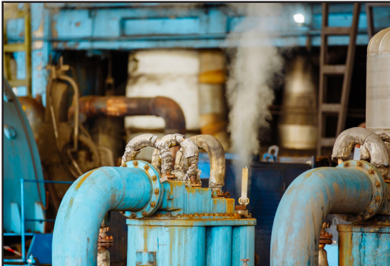
Time-consuming disassembly of flanges on pipes and other equipment.
